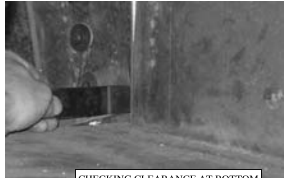
CHECKING CLEARANCE AT BOTTOM OF KNIFE ASSEMBLY
